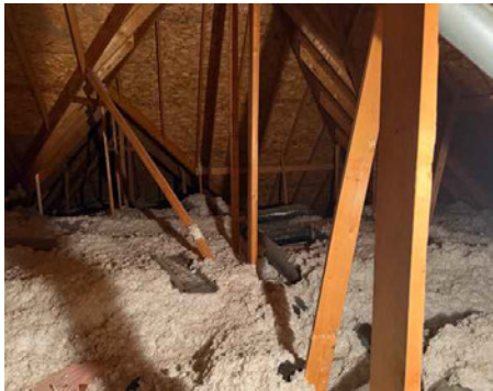
Attic Above 2nd Floor
